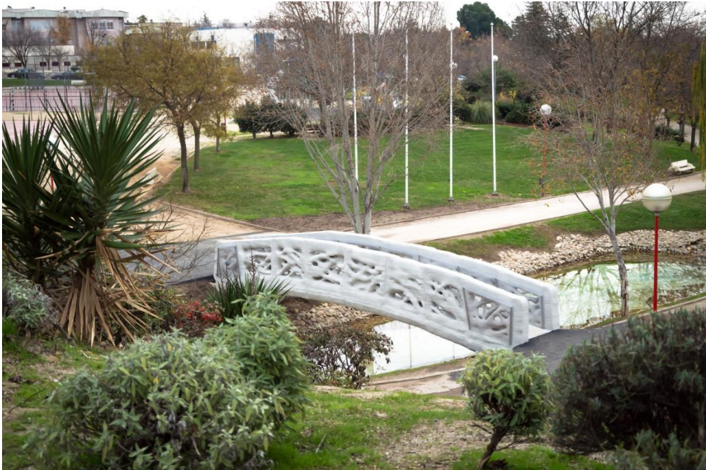
Picture 8. World's first 3D printed bridge - Madrid (Source : [16])
